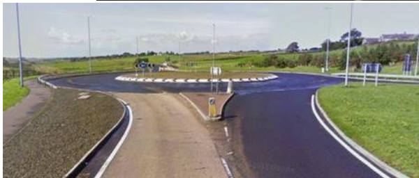
Figure 2 Only Roundabout on the course
