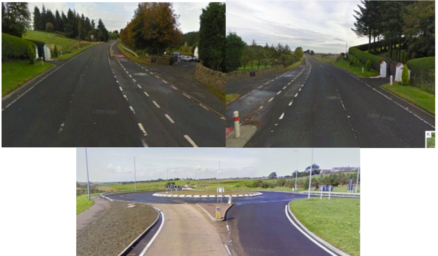
Figure 2 Only Roundabout on the course
